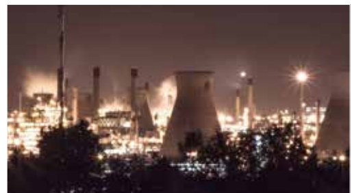
POWER GENERATION FACILITIES
